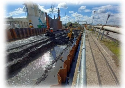
Ridham Stabilisation Works
