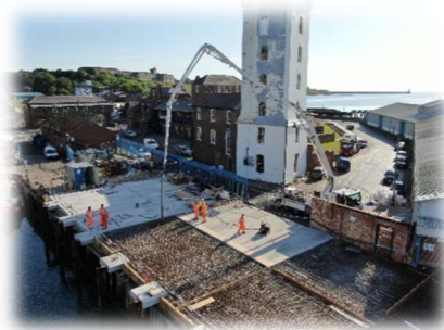
NSFQ Protection Jetty Renewal
