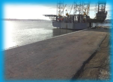
The new quayside facility is one of the strongest in Scotland.
