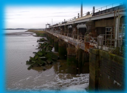
The Weaver Sluices Wave Barrier is a Victorian structure which dates back to the 1890's.
