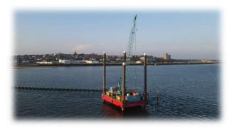
All 3no. Navigation Structures are being constructed from a 250 tonne jack up barge. A significant effort has been made to engage wth the local supply chain in accordance with the councils 'Community Wealth Building Agenda'. Carmet Marine, who are based in the Wirral, were awarded a contract to supply all supporting vessels, and to cordinate the movements of specialist marine plant.
