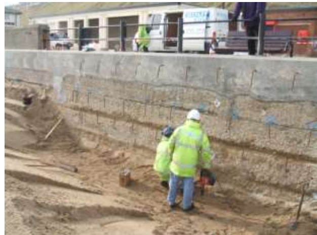
Drilling dowels into the seawall at Marine Walk
