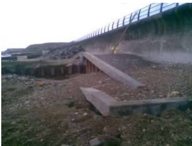
New ramp over the outfall at Hendon
