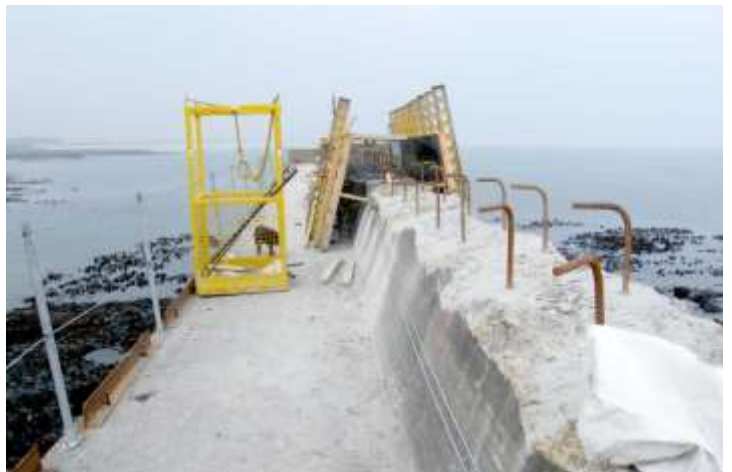
North Breakwater crest repairs
