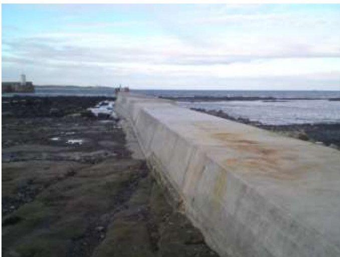
South Breakwater with concrete encasement
