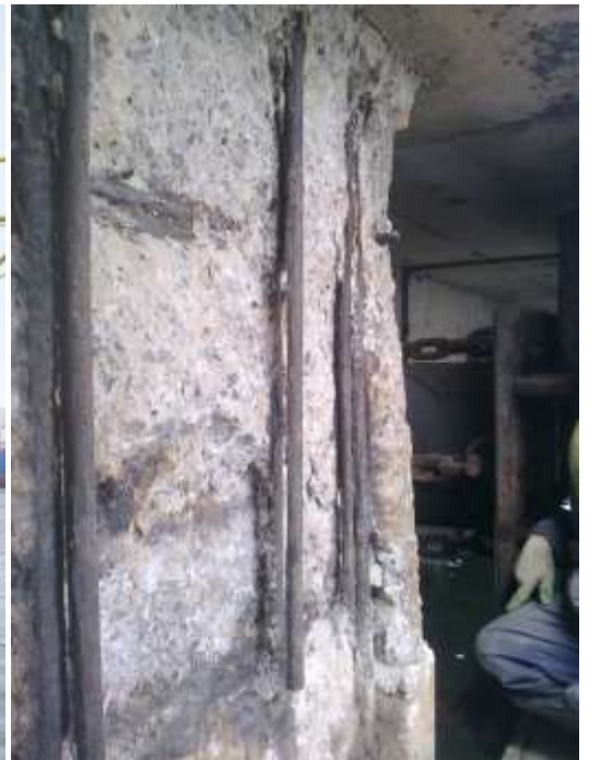
Concrete repairs under jetty
