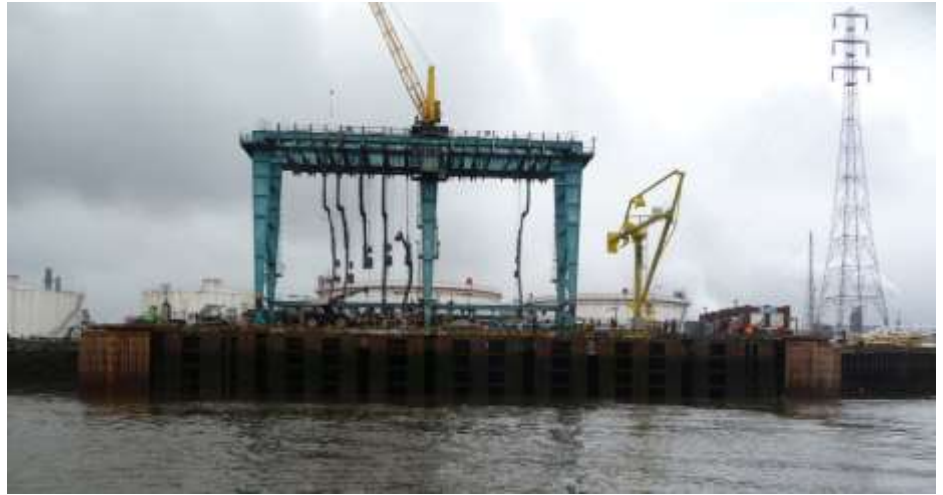
New fenders at east and west of jetty
