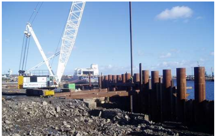
Installation of combi quay wall
