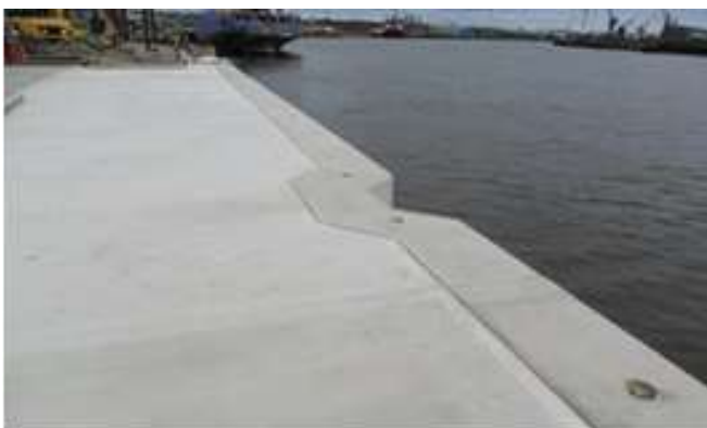
New heavy load out quay.
