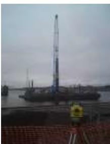
80t crane working off a barge to install mooring piles
