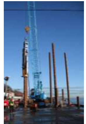
406mm dia tubes driven by hydraulic hammer through the existing deck
