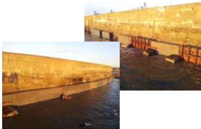
Construction Nearing Completion
