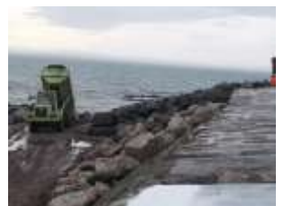
Rock Armour construction during spring tides.
