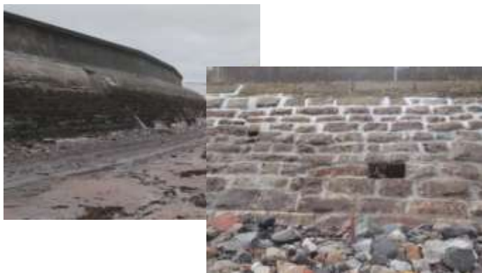
Removal of Marine Growth on Revetment Face
