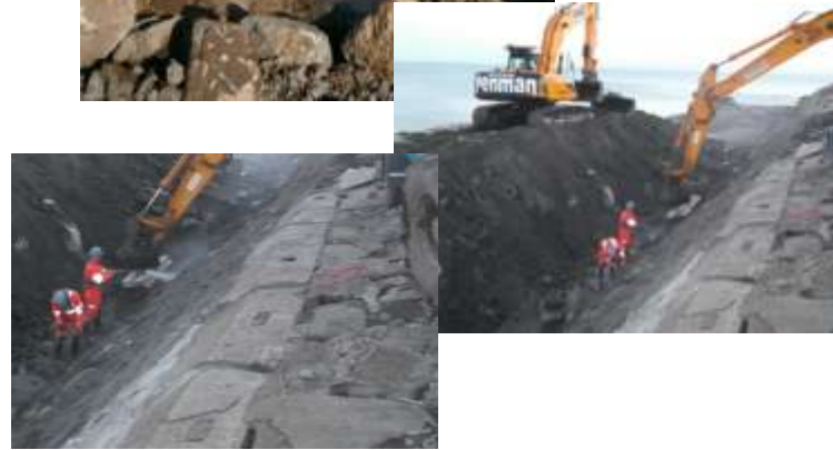
Removal of Marine Growth by Brush Attached to 360 Excavator and High-Pressure Washer
