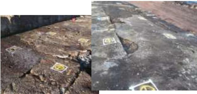
Southbay Civil Engineering sought the specialist drilling contractor, Corecut, to carry out the task of drilling boreholes into the revetment to allow an access for the grout to flow into the revetment.
