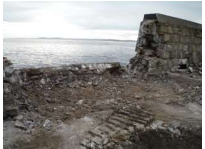
Damaged seawall
