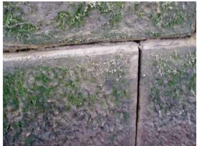
Existing joints cut out for repointing
