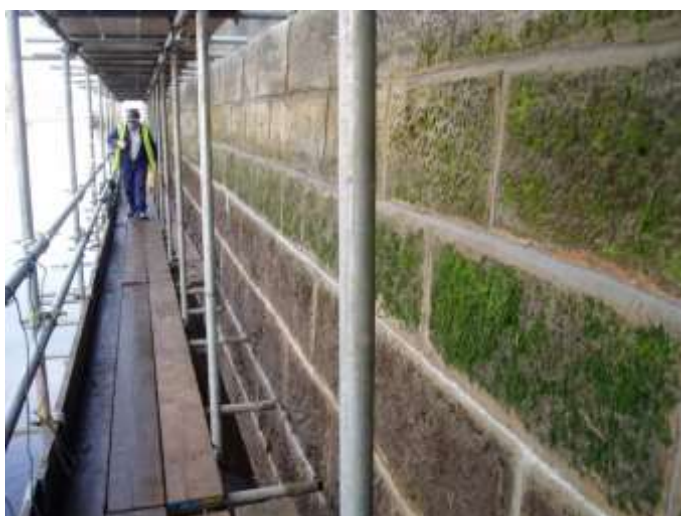
Wall repointed using Easipoint Mortar
