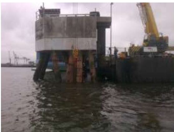
Concrete installed and diving operation underway
