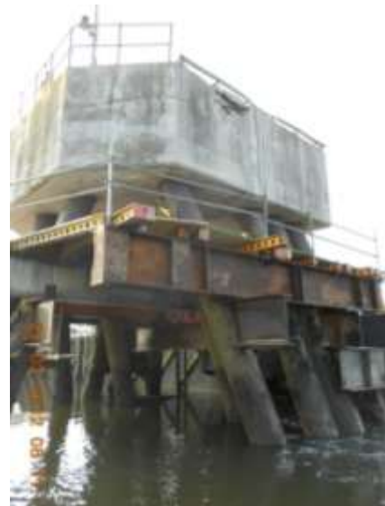
Installation of soffit formwork
