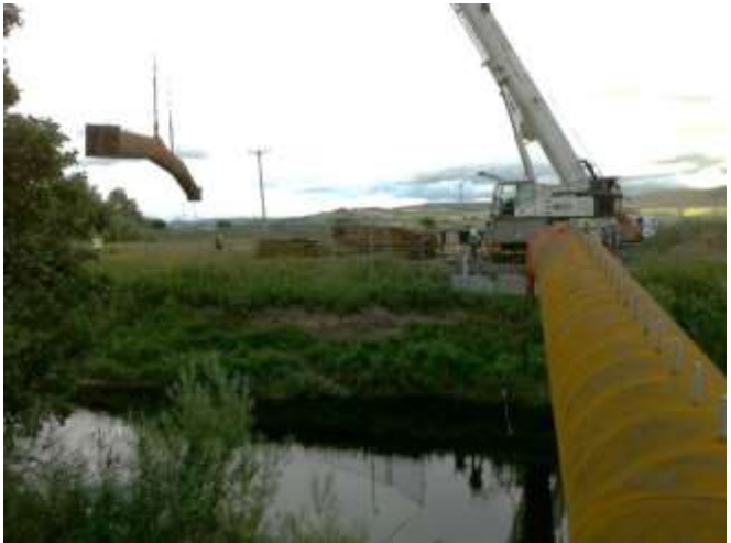
Installation of bridge beams over the River Till
