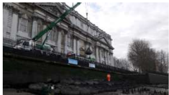
Protection mattress installation via crane
