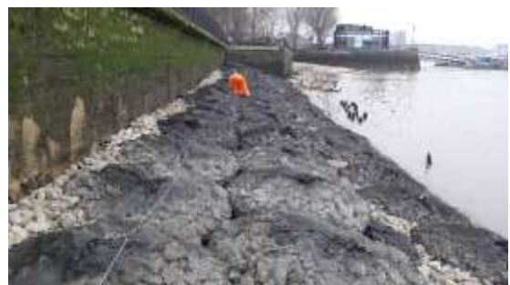
Protection mattresses secured together and voids filled with loose rock
