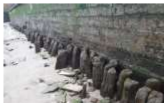
Foreshore erosion exposing Tudor piles
