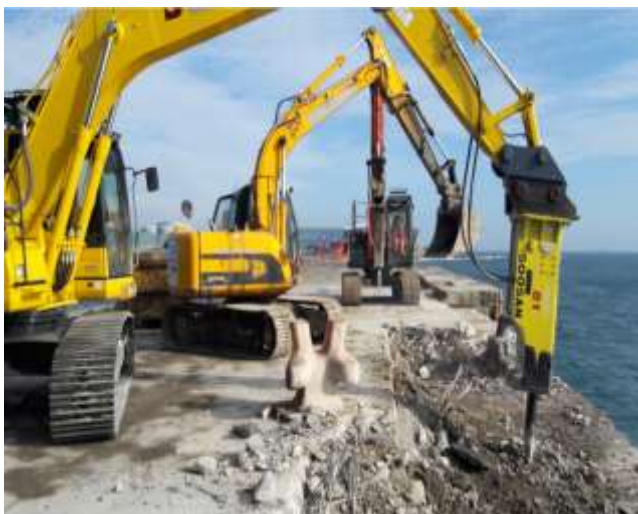
Breakout of the existing damaged section
