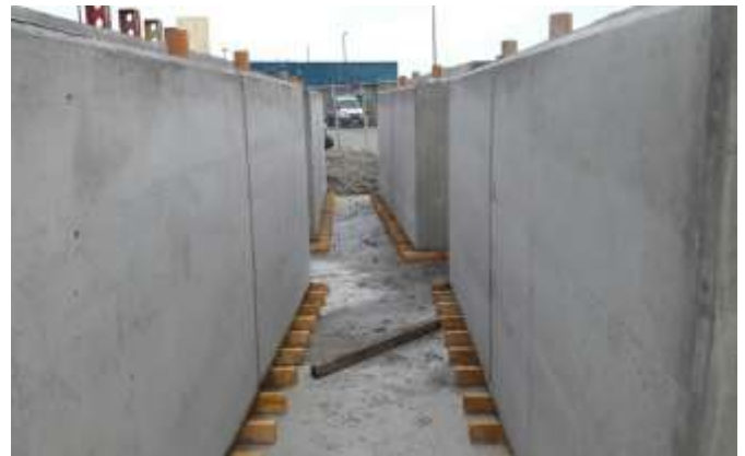
Precast Concrete blocks constructed on site
