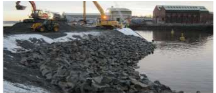
Underlayer Rock Armour Construction with diver assistance
