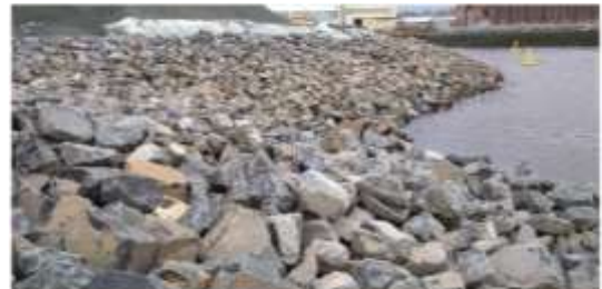
Underlayer Rock Armour Construction with diver assistance
