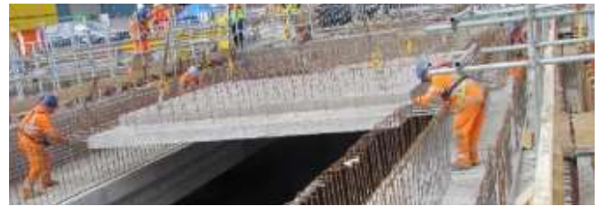
PCC Beams and Planks being placed onto deck extension
