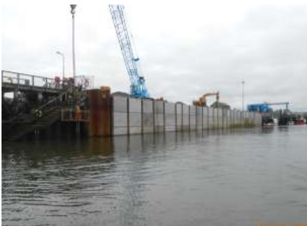
Completed Quay Wall
