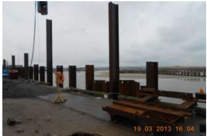
H-Pile / Sheet pile installation
