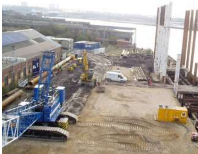
Construction of the ground bearing slab
