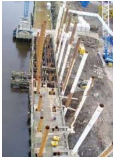
916mm dia steel tubular piles driven into the underlying rock
